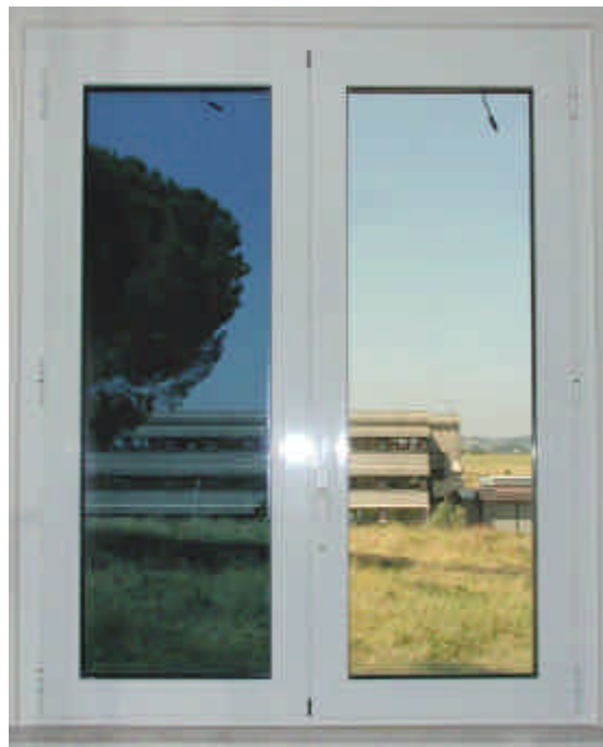
Figure 1 Electrochromic window at ENEA experimental building
